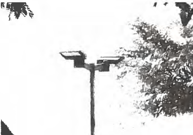
Blow up of photo from patio showing angled up brackets and exposed light fixtures on North Tennis Courts.
